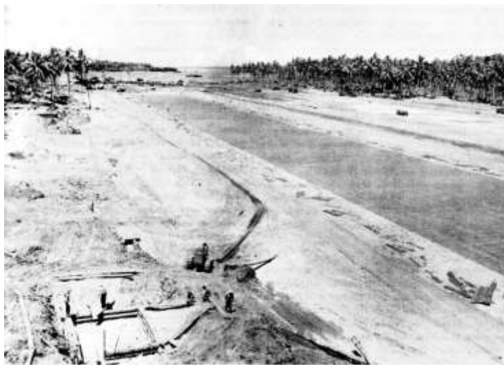
Completed Marston mat airstrip
